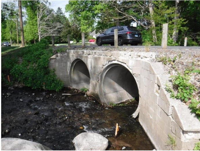
Upstream View – Deteriorated Walls (Pre-Flood)
