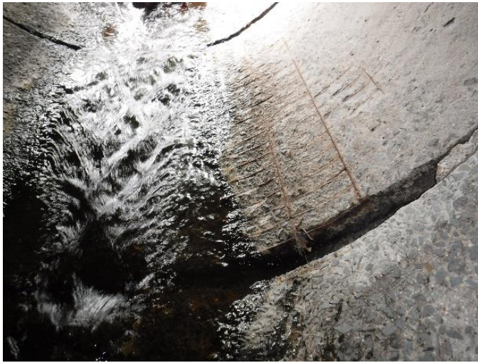
Exposed Reinforcing
