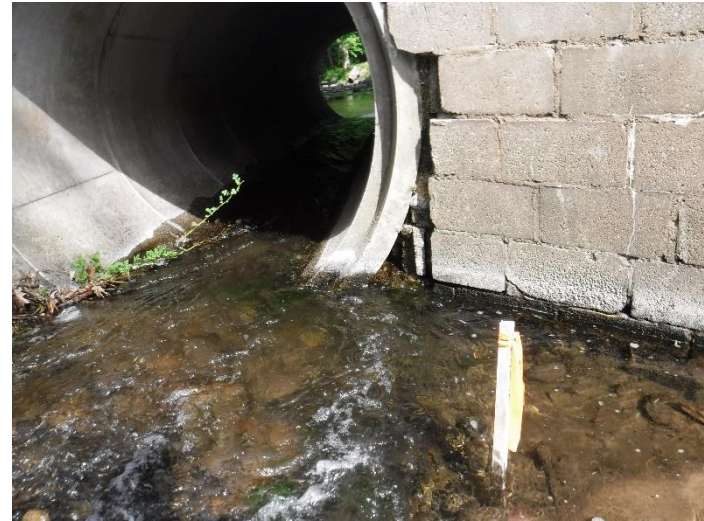
Barrel-Wall Separation with Waterline Scaling (Pre-Flood)
