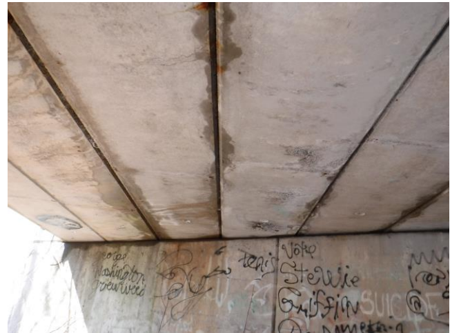
Deteriorated Concrete – Underside of Structure
