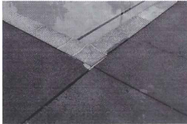
Figure 9 - Wading pool expansion joints
