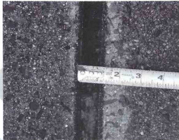
Figure 5 - Deteriorated Expansion Joint
