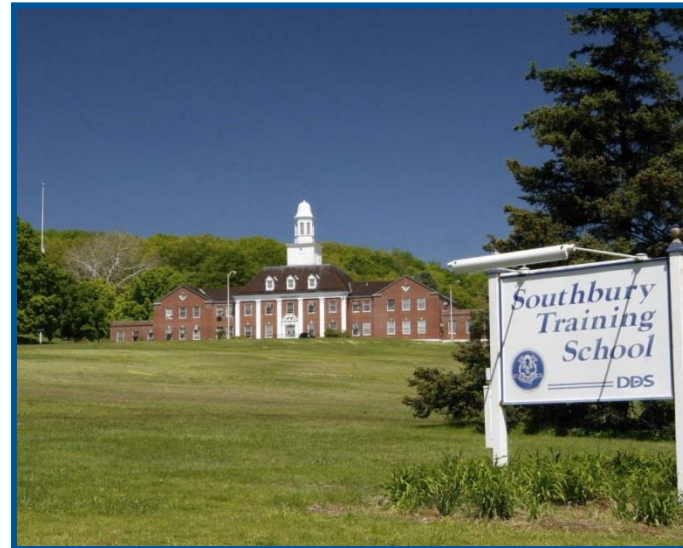
Administration Building and Signage
