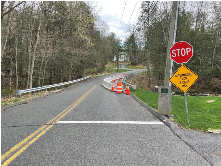
Purchase Brook Road (looking South)
