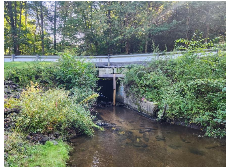
Downstream Culvert Elevation (looking East)
