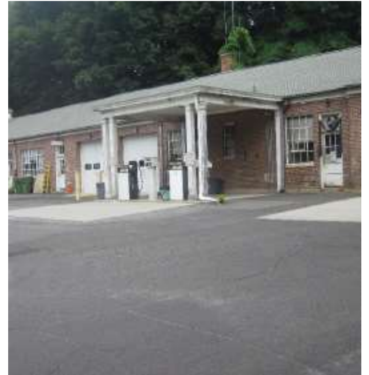
The Phase II ESI recommends additional sampling to test for petroleum release from the underground fuel storage tanks at the maintenance facility building
