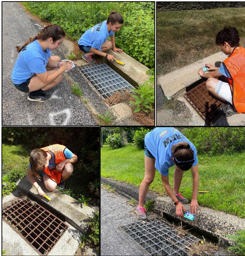
PRWC Summer Interns installing storm drain markers through the Pomperaug Watershed
