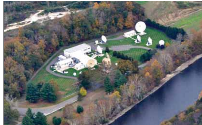
Vizada is a major satellite telecommunications facility
