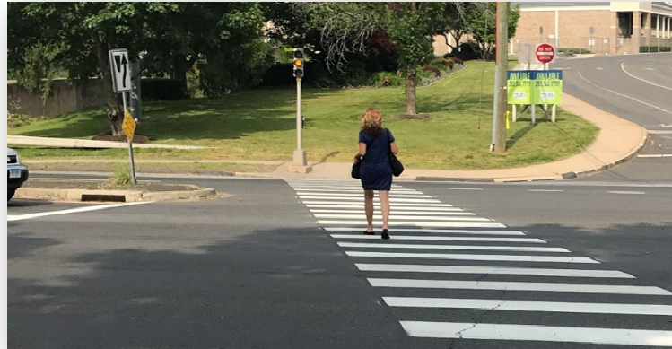
Crosswalk at U.S. Route 6 is without pedestrian countdown signal
