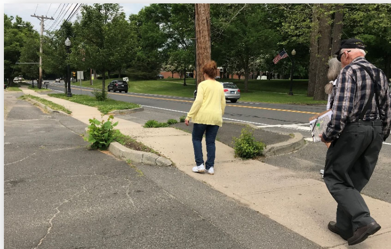
Excessive number of driveway curb cuts, as well as sidewalk up down mogul effect.
